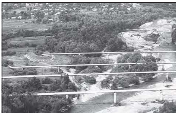
Fig. 8.17: Pipelines transporting natural gas in Ukraine
