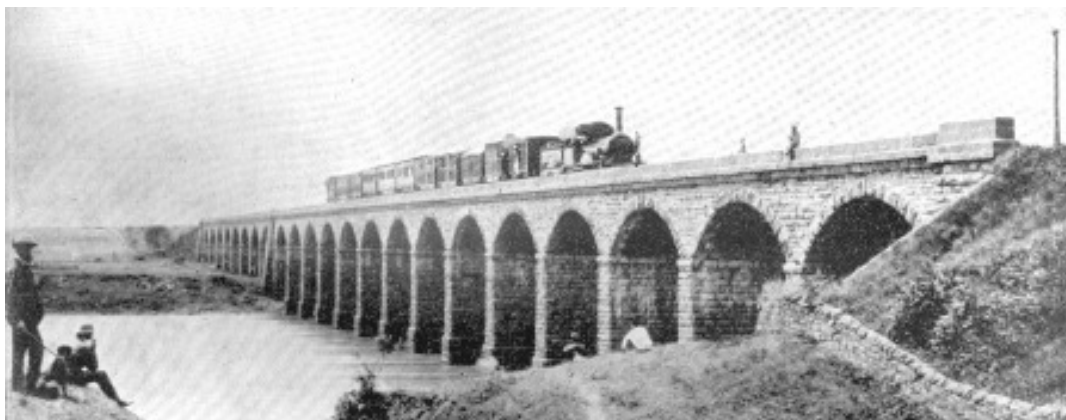
Fig. 1.4 First Railway Bridge linking Bombay with Thane, 1854
